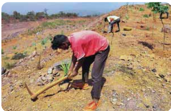
Plantation and contour bunds to control soil erosion
