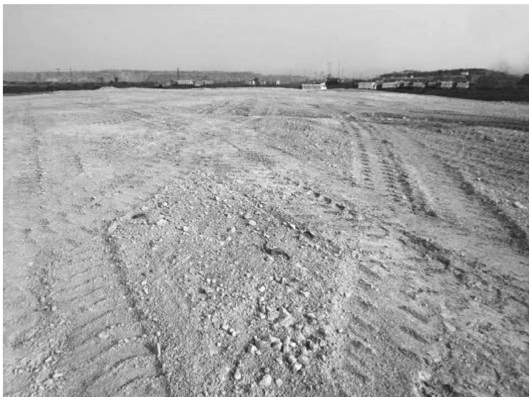
Fig 13. Top soil spreaded evenly on the backfilled quarry
