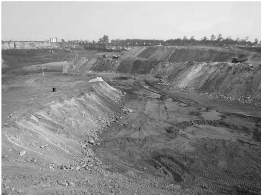
Fig 12. Backfilling of OB in exhausted pilot mine pit
